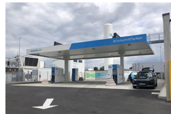
A hydrogen refueling station for local production and consumption in Germany that is the largest in Europe
