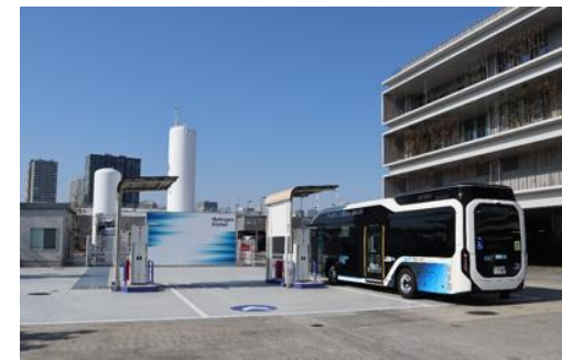
Hydrogen refueling station
