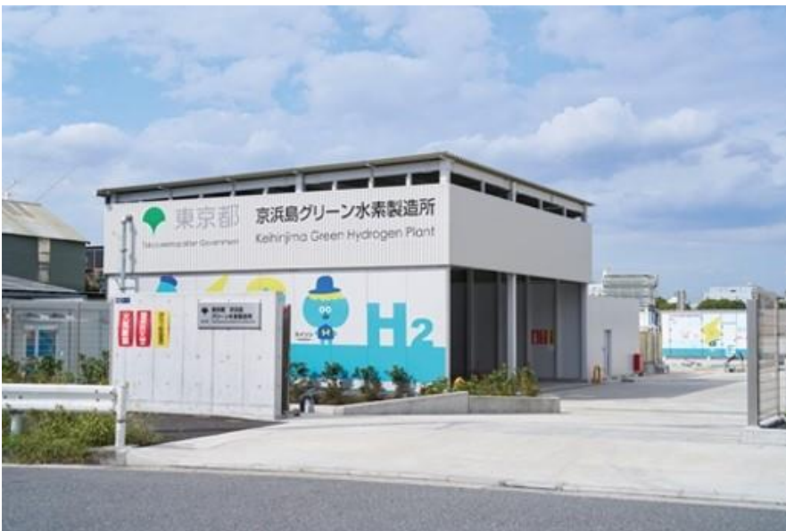
Keihinjima Green Hydrogen Plant
