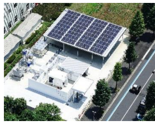
Green Hydrogen Facility © Toshiba Energy Systems & Solutions Corporation
